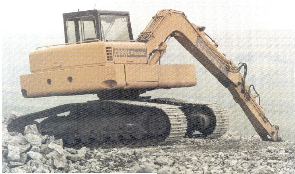
Digger at work in Horton Quarry, England
